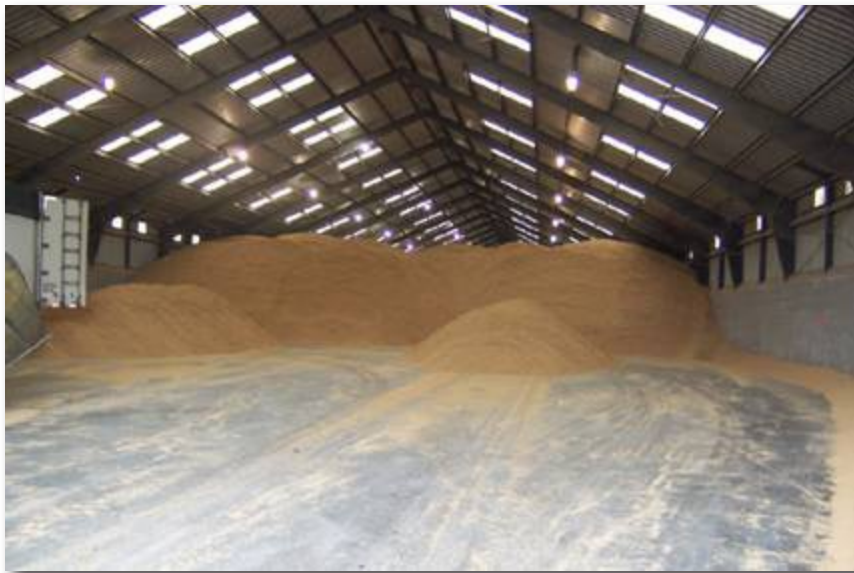
RiceLand Rice Hulls storage facility.
